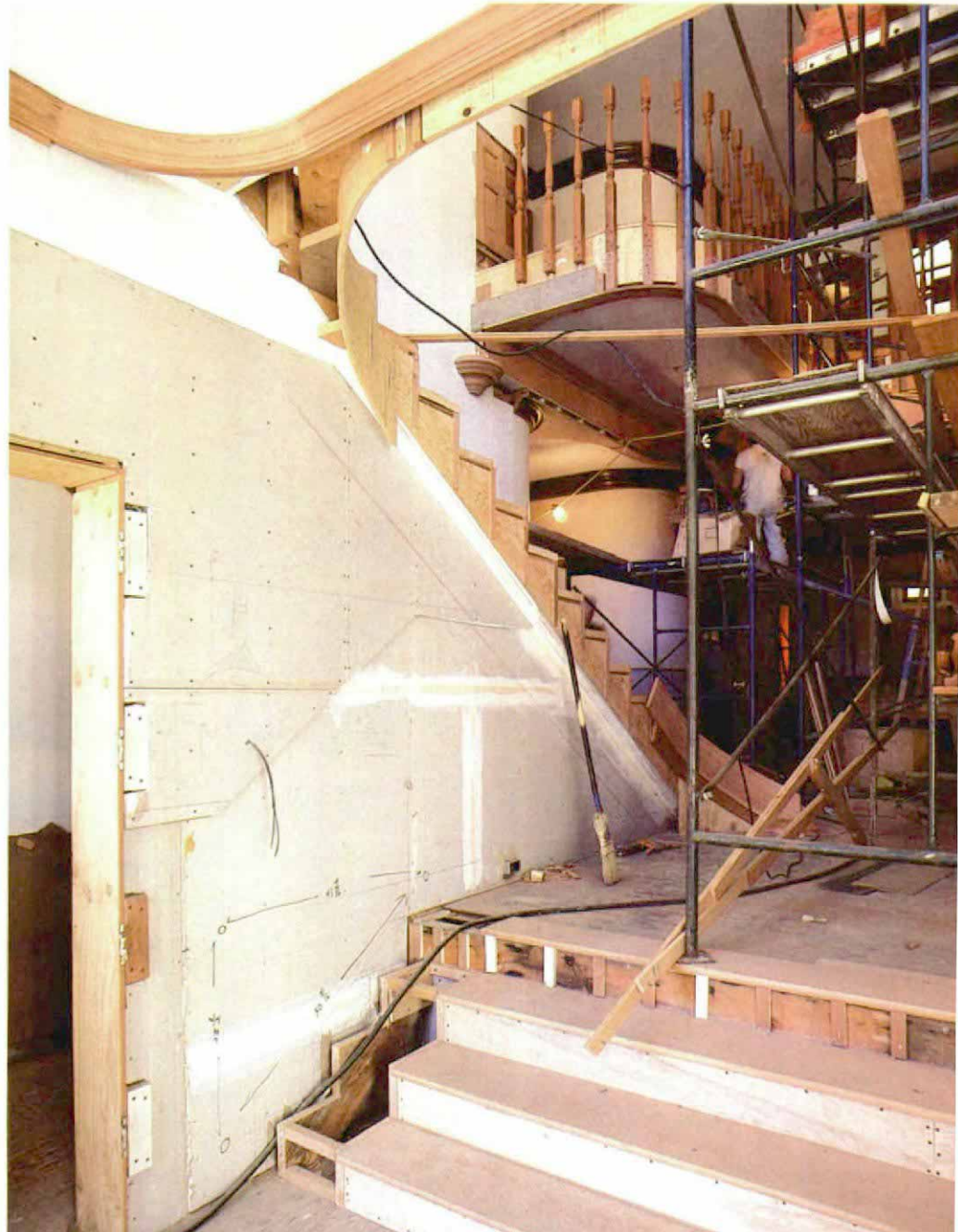
To anchor the formal casings, plywood blocks, seen on the right edge of the door in the photo below, were screwed to the stud wall and the drywall was notched around them. A 1/2-in. plywood nailer was then screwed to the blocks to provide solid backing for the 7 1/2-in. wide door casings, as shown in the drawing at right.
